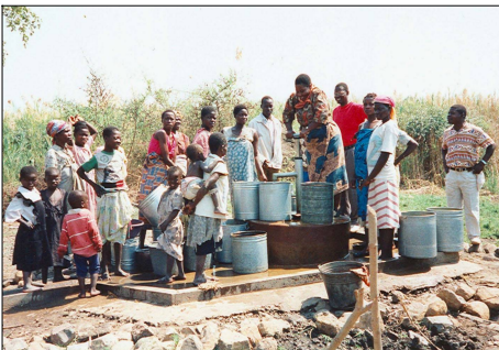
Right: Well at Nsaliva Village with Afridev Pump and Washing Block
