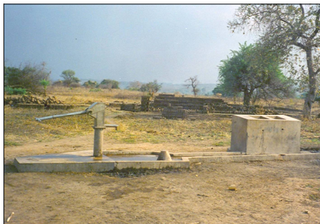
Right: Well at Nsaliva Village with Afridev Pump and Washing Block
