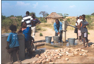
We provide resources what are purchased locally. Our wells use Afridev pumps, the parts for which can be purchased in local markets.
